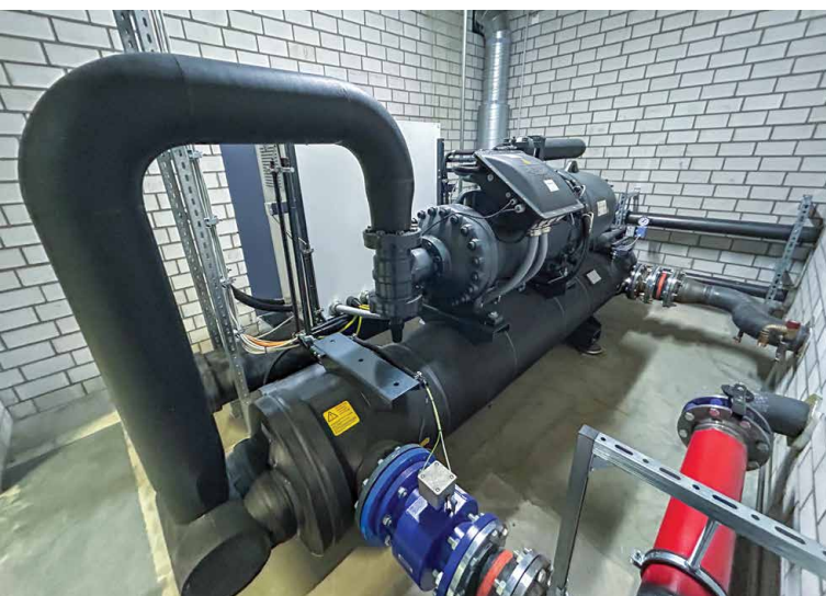
+ Central unit: the new heat pump. With a thermal output of 622 kW, it is 75 times more powerful than a standard heat pump in a detached house.
